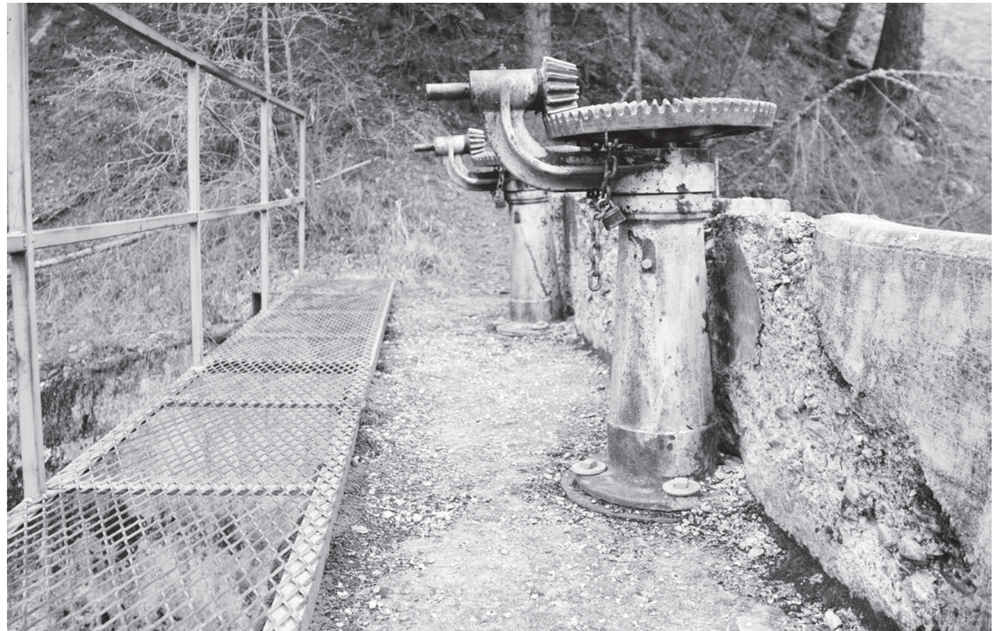
The Flathead Irrigation Project is more than 100 years old. Brumblines and cracked cement can be seen in many areas across the irrigation project. Proponents of the water compact said funds for improvement will come now that Senate Bill 262 has passed.
