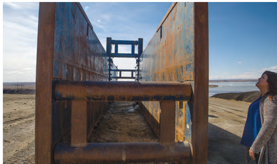
Shalee Russette, project manager for the Rocky Boy's/North Central Montana Regional Water System Project, stands beside a 60-foot long trench box that protects employees working on the pipeline..
