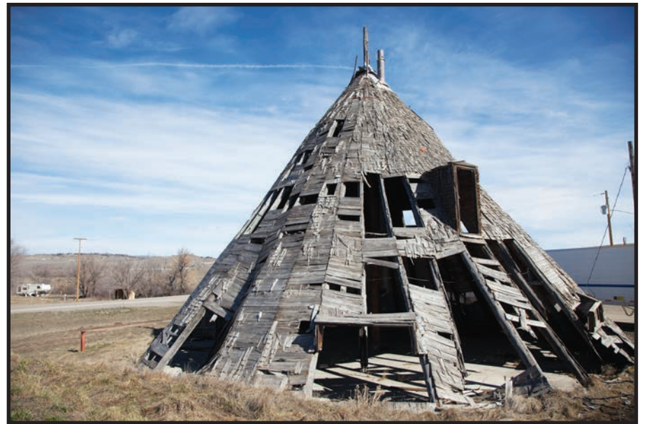
ONE OF THREE wooden teepees built in 1931 still stands in Busby. Major Robinson, an architect, was invited by the residents of Busby to help make a master plan to renovate the structure and make it part of a new campground that will be called Custer's Last Camp.
